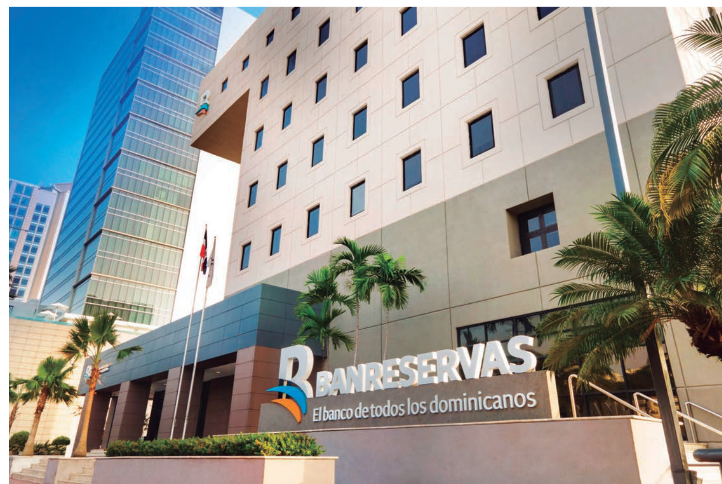
Headquarters of Banreservas in Santo Domingo, Dominican Republic.
